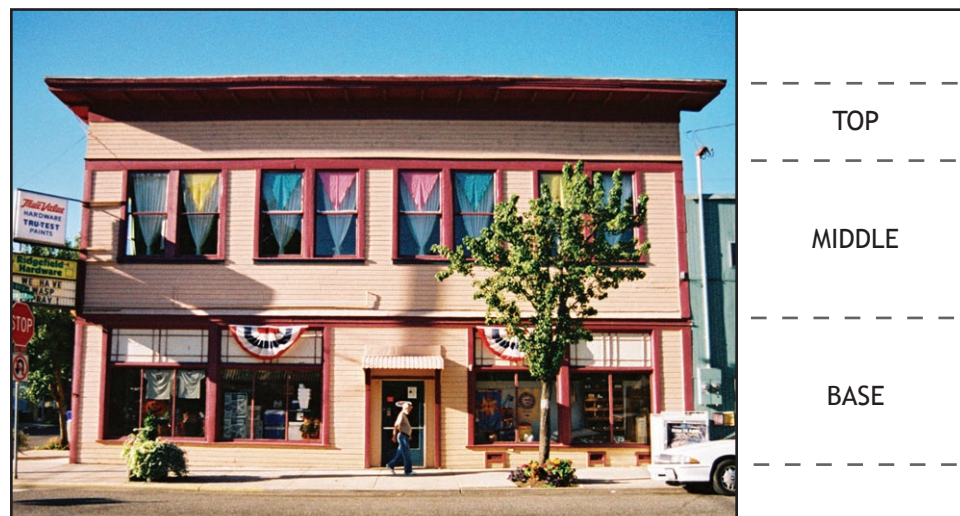
The Hardware store demarcates base and body through simple wood trim bands. The top cornice is formed from a wood trim band, a plain entablature, and a wooden bracketed overhang.
